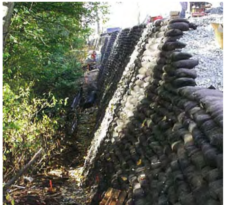
Deltalok during construction
